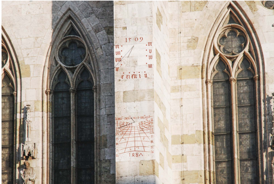
Illustration 1: St. Peter's Cathedral in Regensburg, detail from the south face. The various building materials used in the facade are clearly evident: the darker, somewhat green stones are the original sandstone, while the lighter stones are more recent limestone replacements. Photograph taken by the author in 2008.
